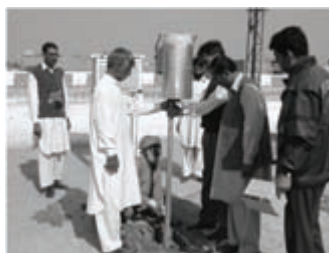
Fixing of Wet-Only Collector
