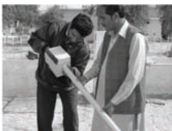
Fixing of Bulk Collector
